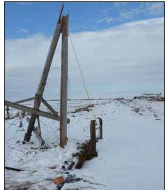
Line crews work to restore damaged poles following the Nov. 16 snowstorm.
