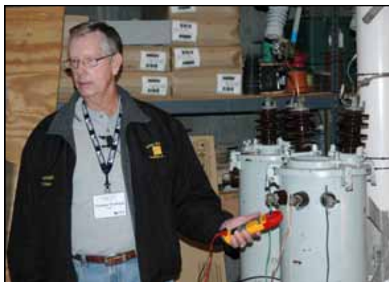
Norm McDugle, OAE, talks about single-and-three-phase load calculations at the transformer workshop.
