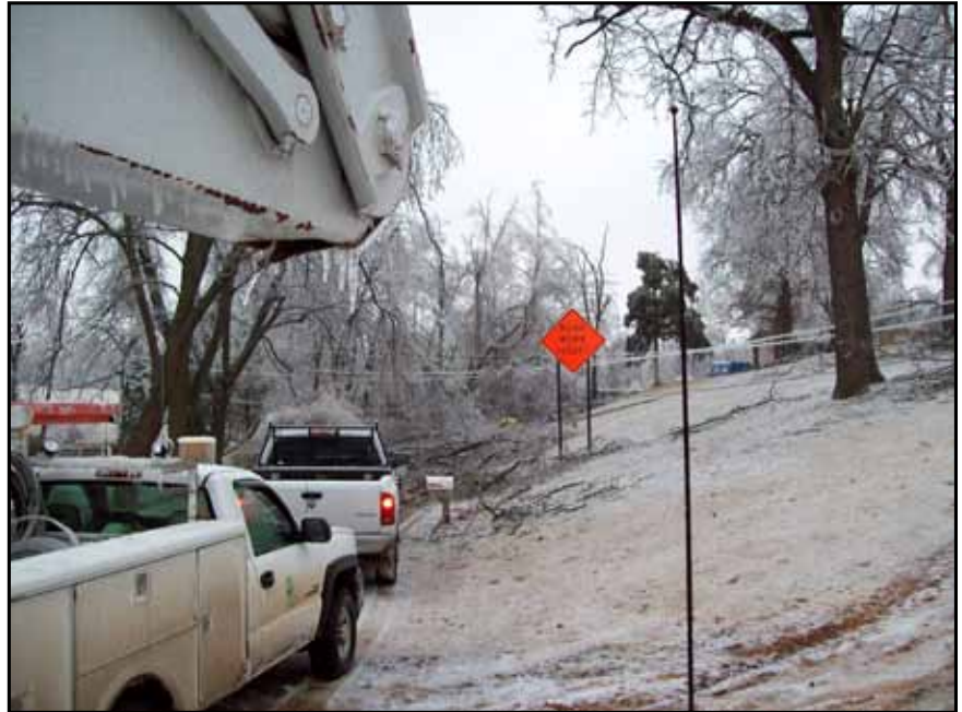
Snapped utility poles, fallen trees, and downed lines make the storm recovery efforts challenging for the line crews in Arkansas.
