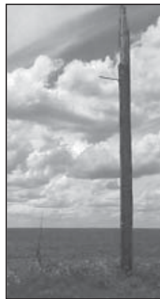
A lone splinter stands where an "H" fixture once held a transmission line.
