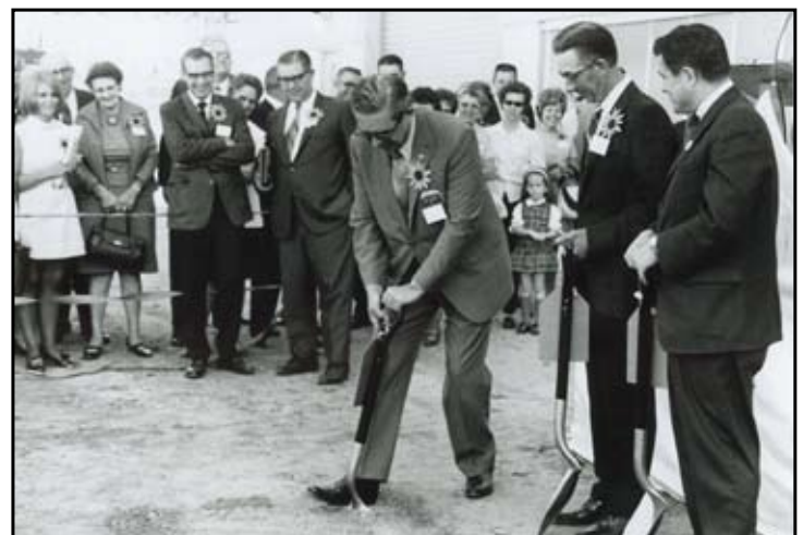
Officials break ground in 1970 for the new S-2 plant. From left in the background are Phil Lesh and Dale Saffels of the KCC. With the shovels are a representative from REA, Sunflower’s president Wilmot Price, and Gov. Robert Docking.
