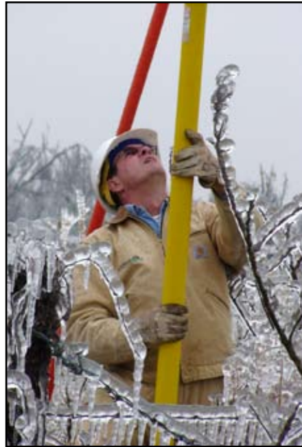
Heartland lineman, Jerry Cochran, repairs lines during the 2007 ice storm.
