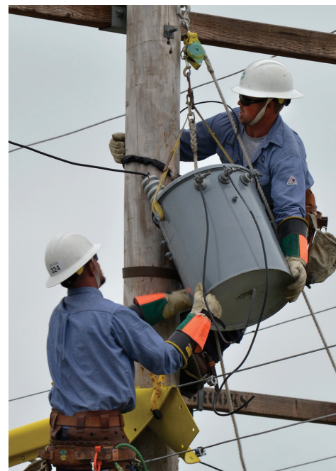
The Hays Journeyman team of Brian Legleiter and Butch Hamel detaches a transformer, as Groundman Daniel Hodges lowers it. The Hays team placed in the top third overall.
